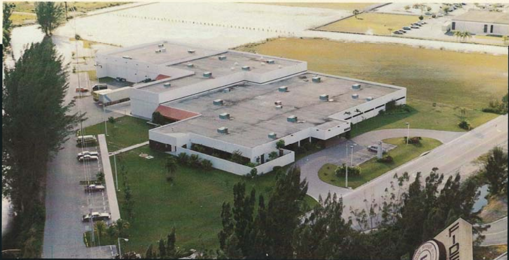
Main Plant Facility on 12 acres.
